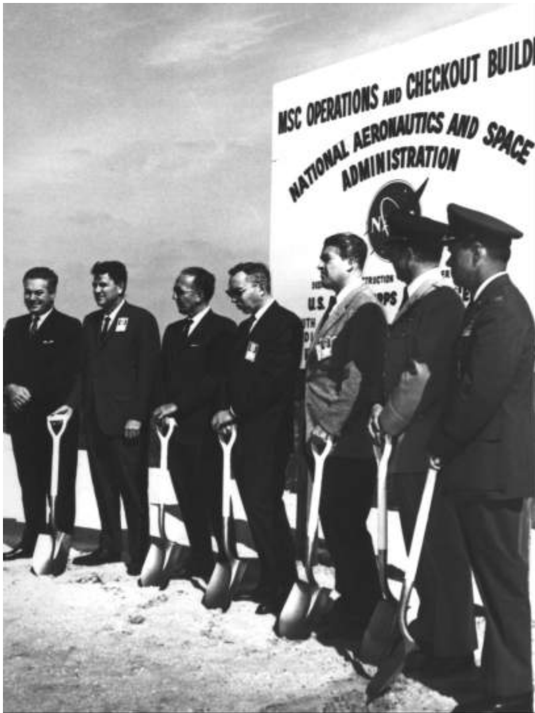
Ground was broken for the MSC Operations and Checkout Building at Merritt Island January 28, 1963. Participants were, left to right, Walter C. Williams, Director of Flight Operations, MSC; G. Merritt Preston, Director of Pre-Flight Operations Division, MSC; Kurt H. Debus, Director, Launch Operations Center; D. Brainerd Holmes, Director, NASA Office of Manned Space Flight; Wernher von Braun, Marshall Space Flight Center; Col. H. R. Parfitt, District Engineer, U.S. Army; and Col. E. Richardson, U.S. Air Force.
