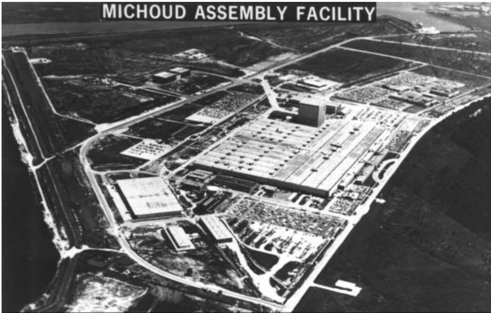
Aerial view of the Michoud Operations Plant, New Orleans, La
