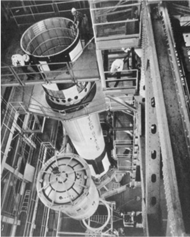
Figure 91. Second stage of Gemini launch vehicle 5 being hoisted to the top of the vertical test facility at Martin-Baltimore. (NASA Photo S-65-2867, Feb. 8, 1965.)
