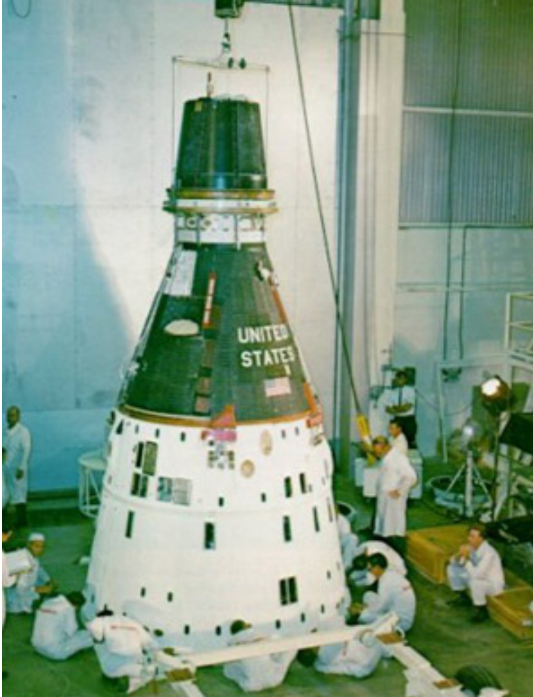
Figure 126. McDonnell personnel bolting the Gemini XI spacecraft to a support ring for boresighting in the Pyrotechnic Installation Building, Merritt Island. (NASA Photo S-66-47635, July 2, 1966.)
